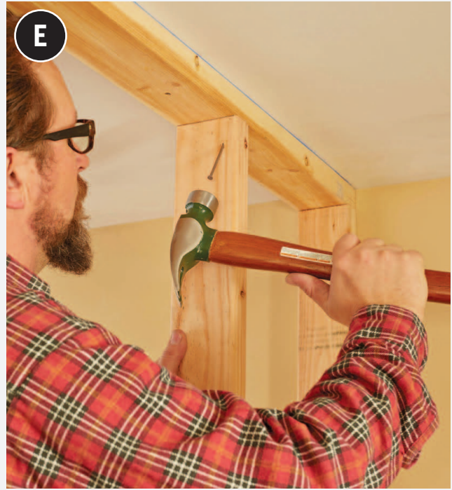
Position the loose ends of the studs against the top plate following the reference lines and then toenail the studs to the plate.
