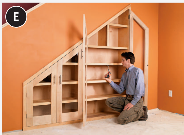
Cover the gaps between the new project and the old wall surface with wood trim.
