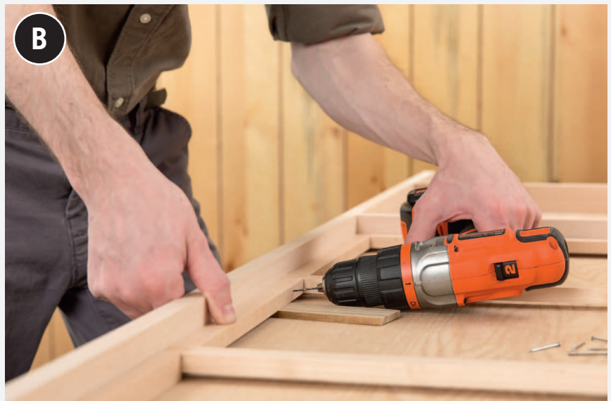
Drive pilot holes for all screws and brads , including those attaching the vertical retainers to the uprights.
