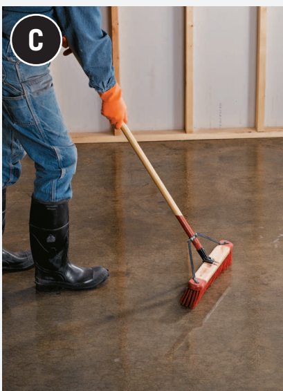
Work the acid solution into the floor with a push broom.
