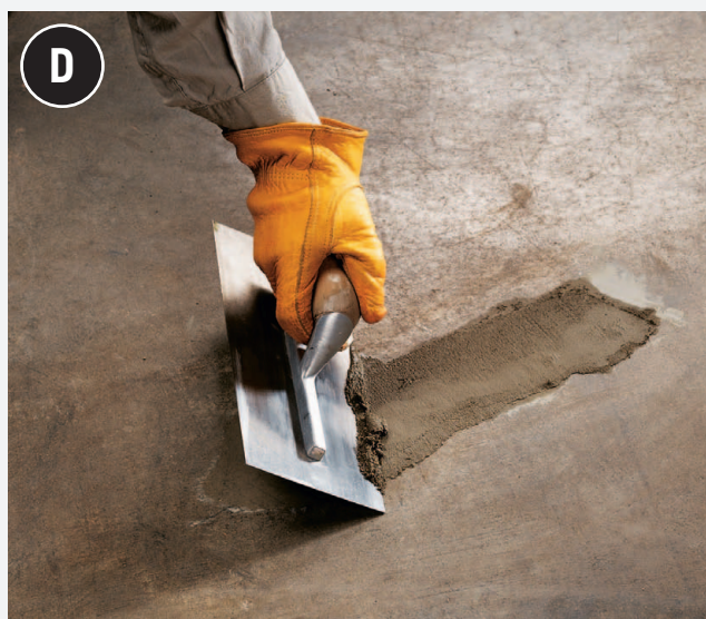
D Pack the repair area with fortified concrete repair compound and then remove excess and smooth the surface with a concrete trowel.
