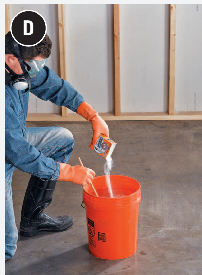
Mix baking soda into water and broom it onto the floor to neutralize the acid after letting the acid work for up to 10 minutes. Rinse well with clean water.
