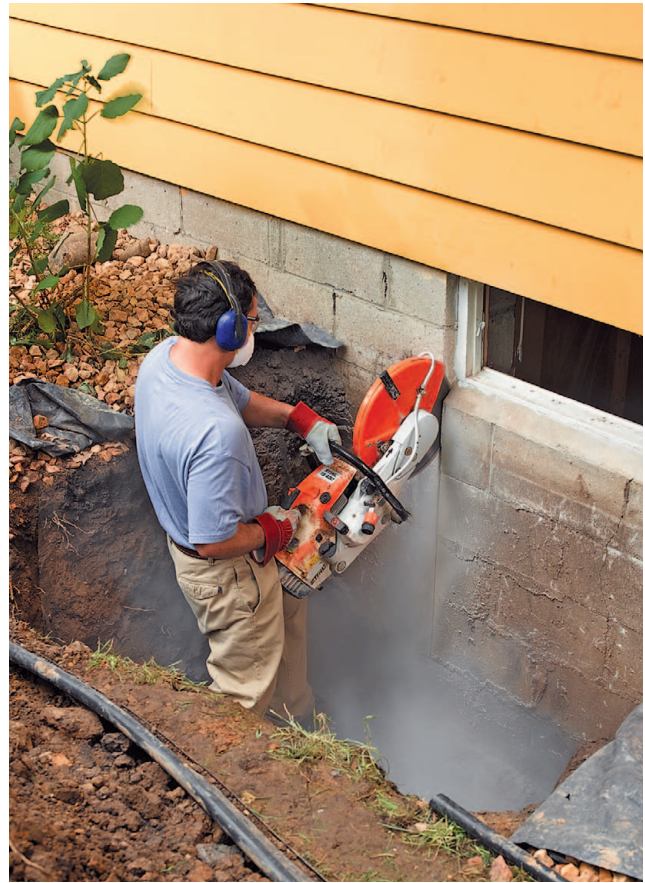
Installing a new window that meets minimum egress rules often means deepening the existing window opening by removing a section of the masonry foundation wall beneath the window opening.
