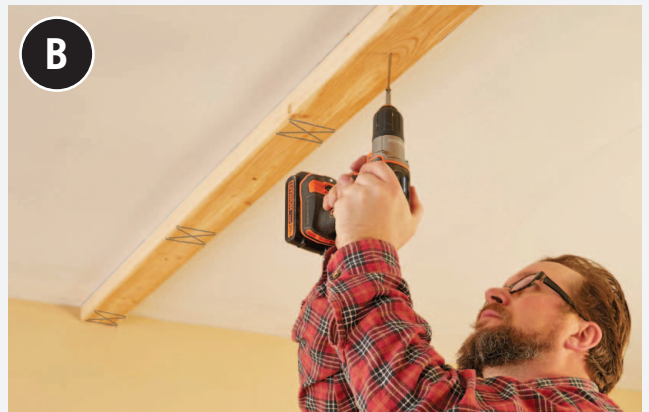
Follow your reference lines to position the plate against the ceiling and attach it at joist locations with construction screws.
