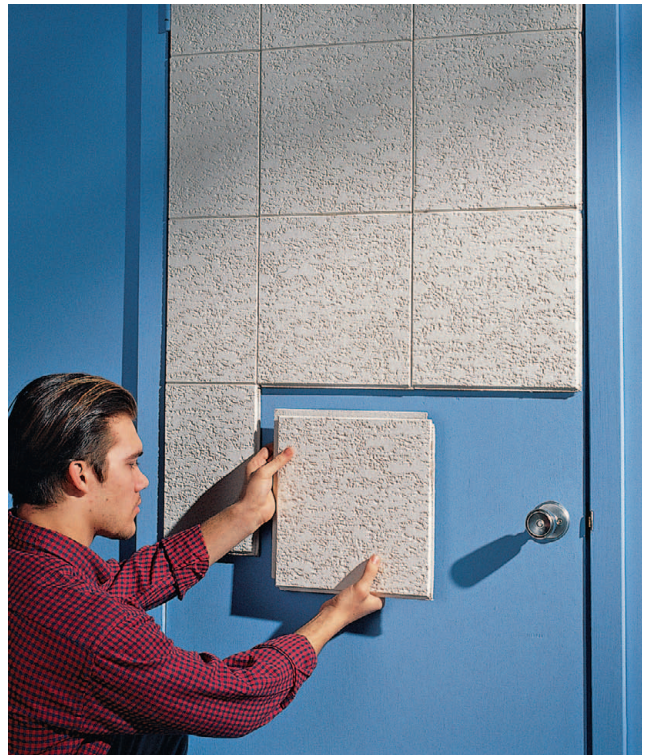
Hanging heavy textiles or affixing acoustical tile to key noise transfer points, such as hollow-core doors, can reduce noise transfer. Solid doors offer a more permanent improvement.
