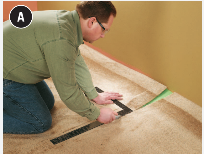
Remove old floorcoverings in the exact installation area to expose the floor sheathing.
