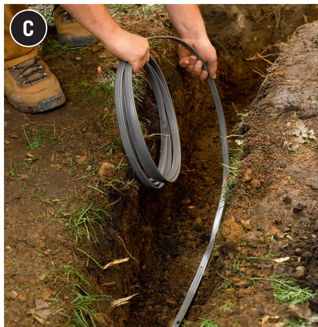
From the L-body fitting , UF cable travels through a trench to reach the outbuilding. The cable should be contiguous, with no splices.
