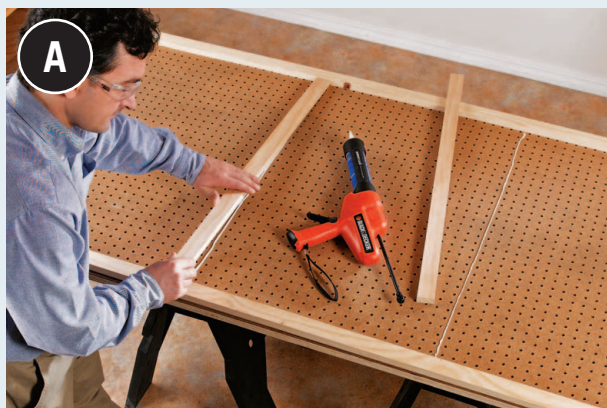
Secure the furring strips with construction glue and screws. Add intermediate vertical furring for extra rigidity.
