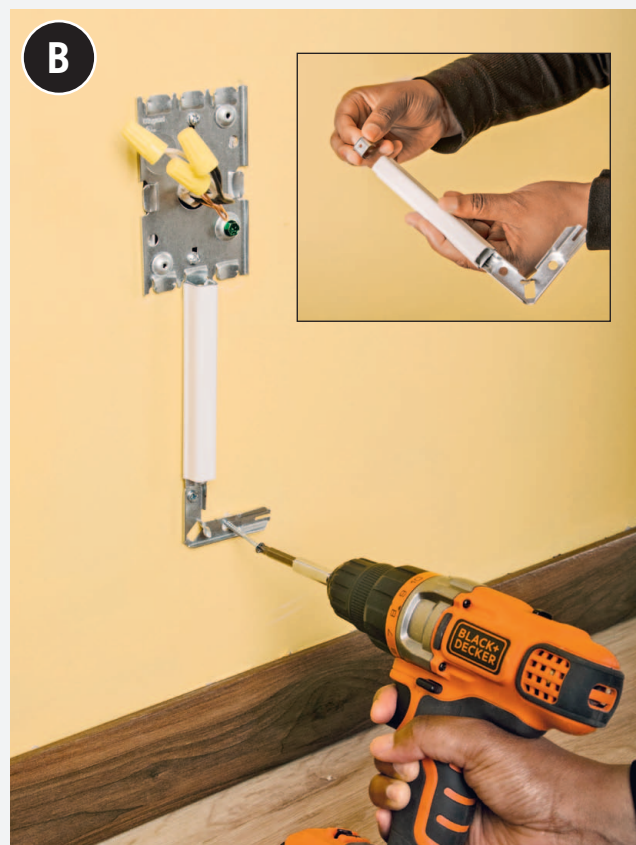
Fit the elbow base into the track section, insert the section into the box, and then attach the elbow base plate on the wall.
