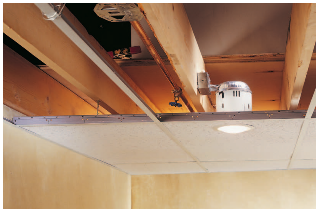
Suspended ceiling hung from wire-supported metal tracks easily integrates with canister lights, ceiling fans, and other ceiling elements and allows access to the joist cavities.
