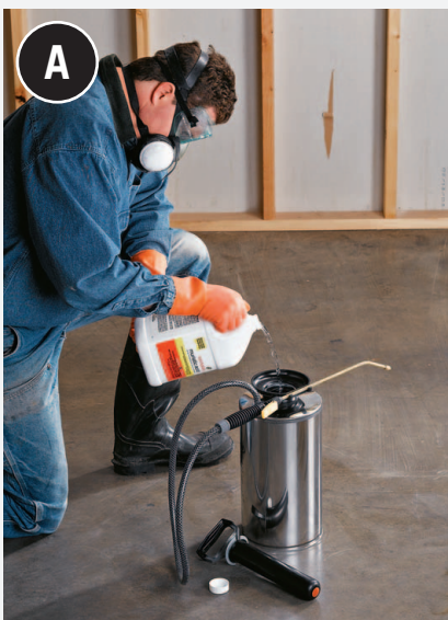
Add the muriatic acid to the water in the sprayer container at a rate of one part acid to three parts water.
