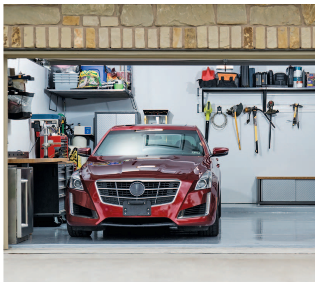
This single LED fixture casts bright, even light throughout the garage while casting minimal shadows.
