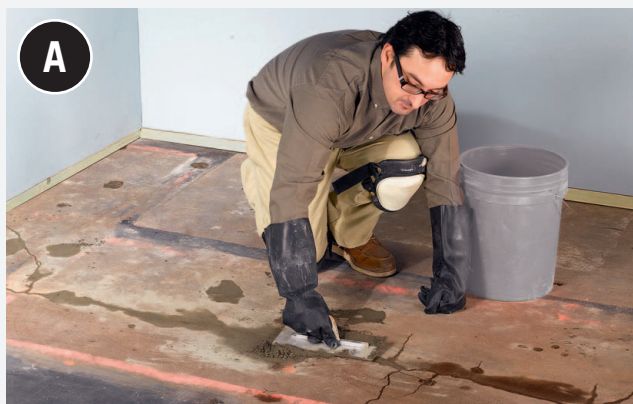
Trowel a stiff mixture of the concrete resurfacer into any holes, divots, or low areas before you pour resurfacer at its regular consistency.
