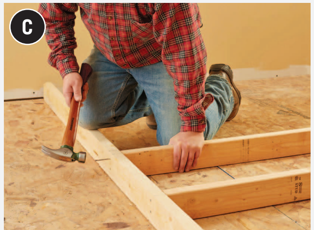
Driving 16d nails through the base plate and into the stud ends is easier and more secure than toenailing the studs after installing the base plate.
