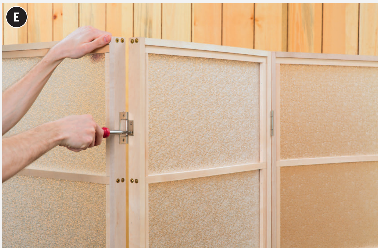
Fasten the room divider panels together with butt or bifold hinges (shown). Apply a topcoat to the wood parts if you wish.
