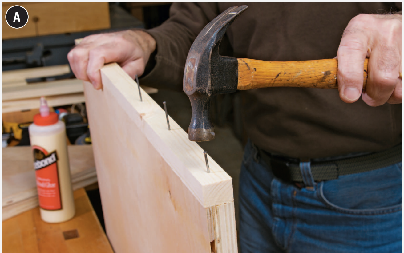
Fasten the edging strips, set the finish nails, and fill in the holes with wood putty
