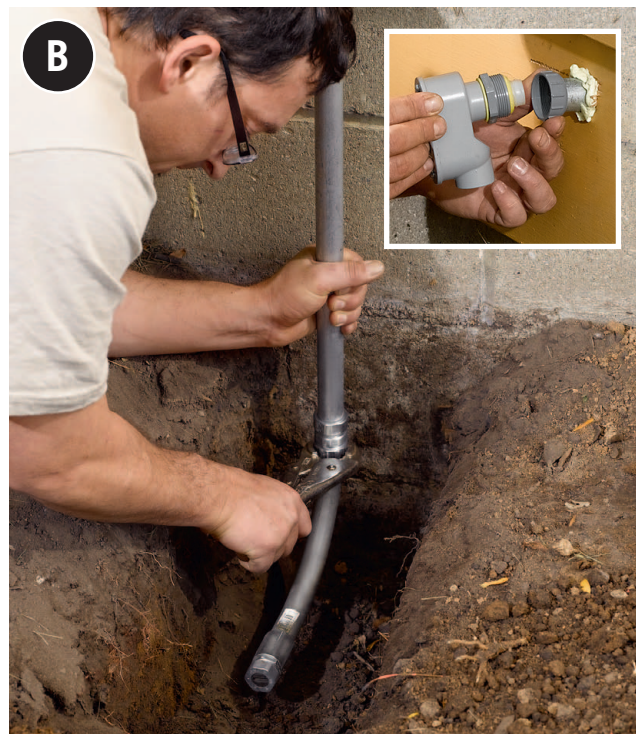
Exterior-rated conduit attaches to an L-body fitting mounted on the house exterior (inset photo), then runs downward to a depth of 12 to 24 inches and attaches to a 90° sweep.
