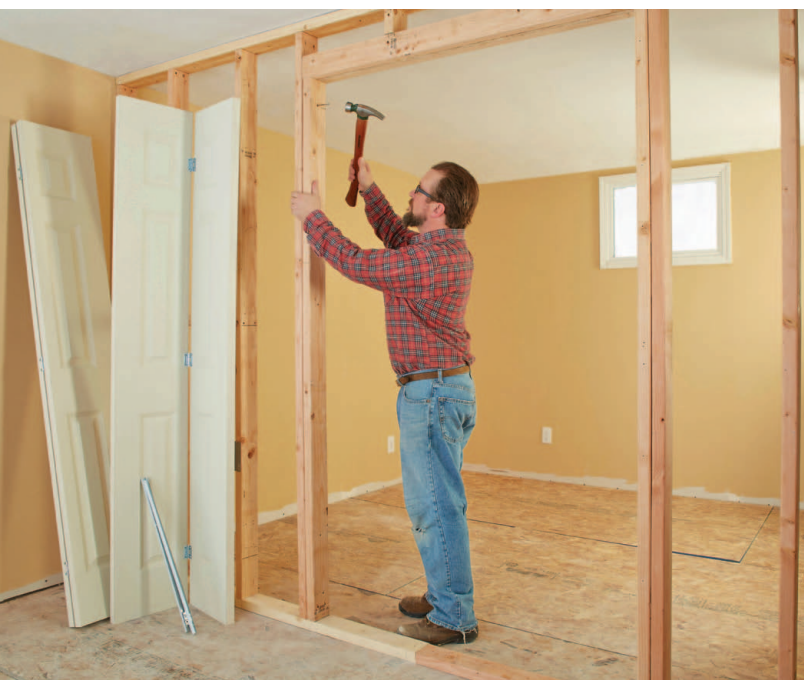
The basement partition wall being framed here has a rough opening for a bifold door instead of a typical passage door.
