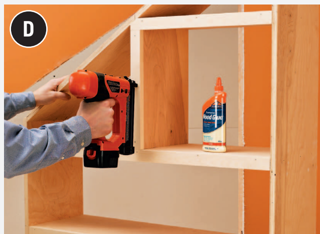
Attach 1 × 2 shelf edging to all exposed edges, butting the edges of the vertical strips against the horizontal ones.
