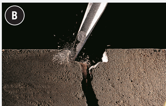
B Use a cold chisel and mallet to taper side walls downward to help keep the repair product from popping out.
