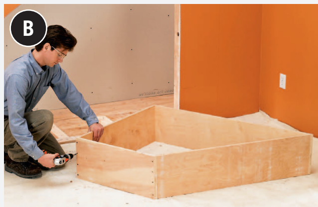
Cut plywood tops, bottoms, and sides for each trapezoidal carcase unit and join the parts with glue and wood screws.
