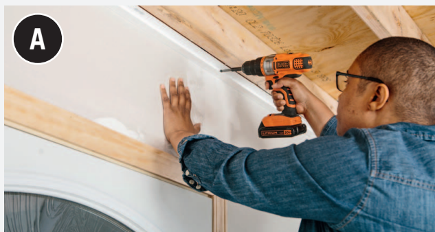
Use drywall screws to attach the U-shaped wall channels at the junction between the top of the wall and the ceiling.
