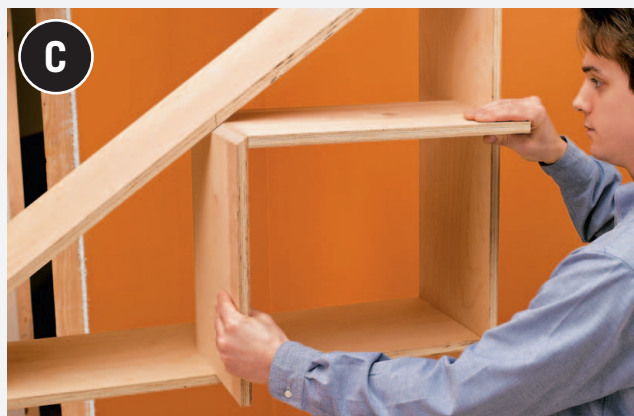
Attach the L-shaped inserts at the tops of the openings.
