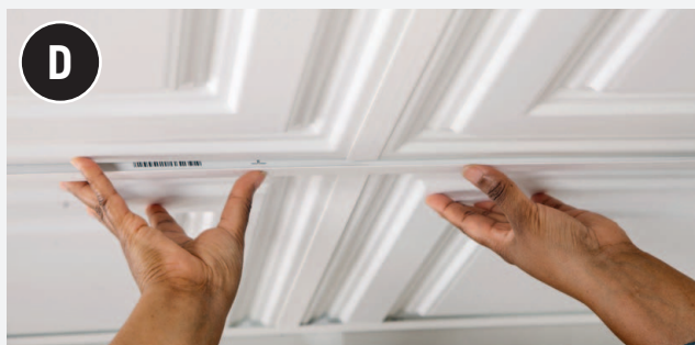
Finish the installation by snapping the runner strips into the slots in the hanger strips.
