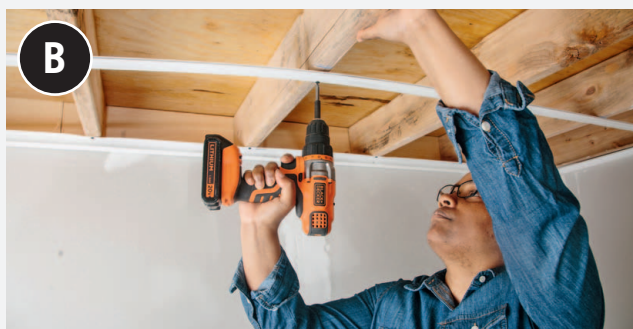
Attach the first row of hanger tracks perpendicular to the ceiling joists, with the ends inserted into the wall channels.
