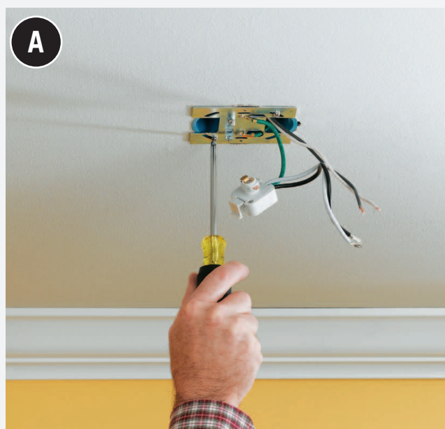
Shut off power , remove the old fixture (or provide a new electrical box with wired hookups), and attach the mounting strap to the electrical box.
