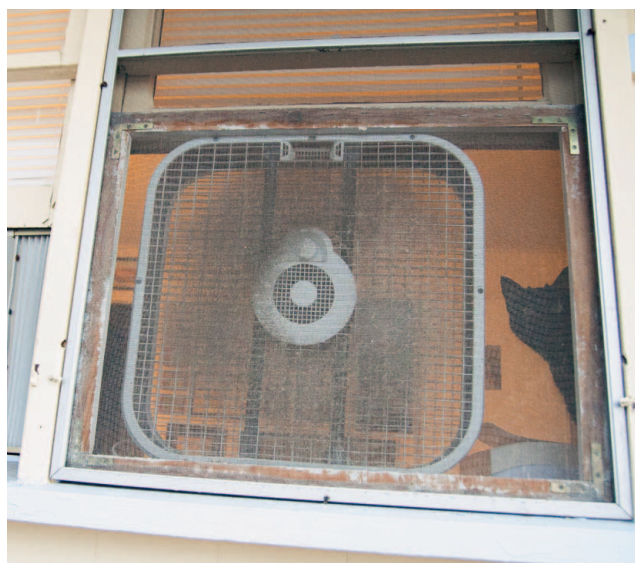
Window-mount fans fit into an existing window opening in much the same way as a window air conditioner to assist in air movement in or out of the room.
