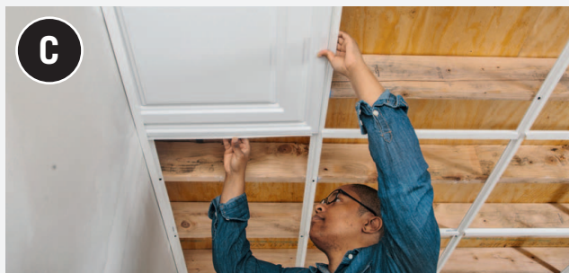
Begin installing the full-size field panels by fitting them into the grid openings so they rest on the hanger track ledges.
