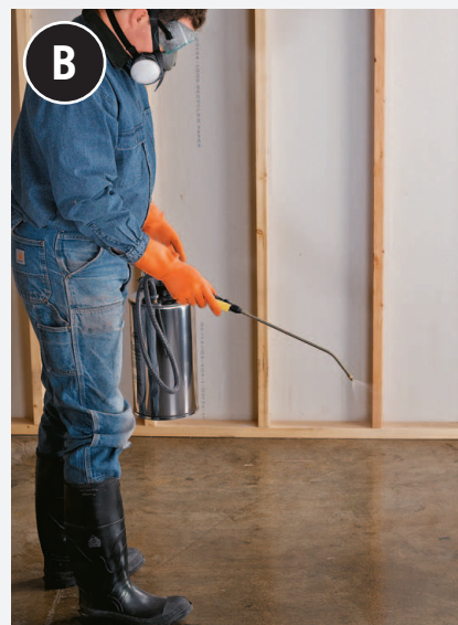
Spay an even coat of acid solution onto the damp concrete floor.
