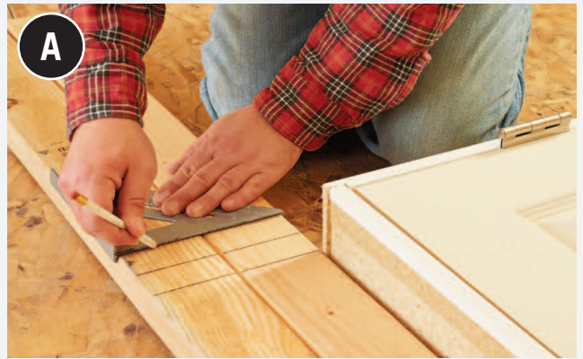
Use a square to gang-mark locations for all studs onto the top and sole plates.
