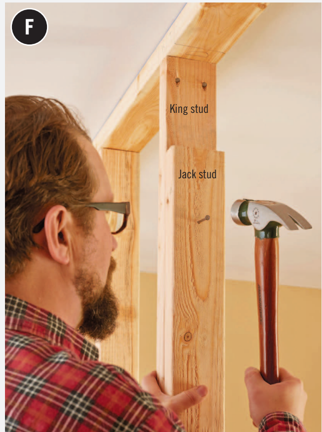
Face-nail the jack studs to the king studs to create a properly dimensioned rough opening for your door.
