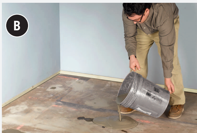
Work in 100-sq.-ft. sections when pouring the resurfacer mix.
