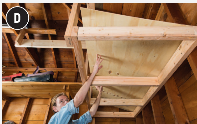
D Cut a plywood platform and slide it in place.
