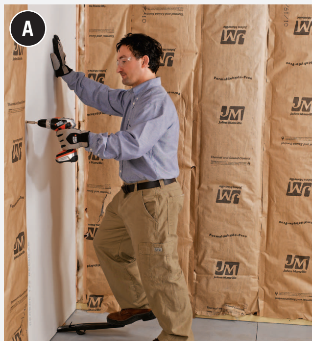
Use a drywall lifter to raise the panels off the floor as you attach them.
