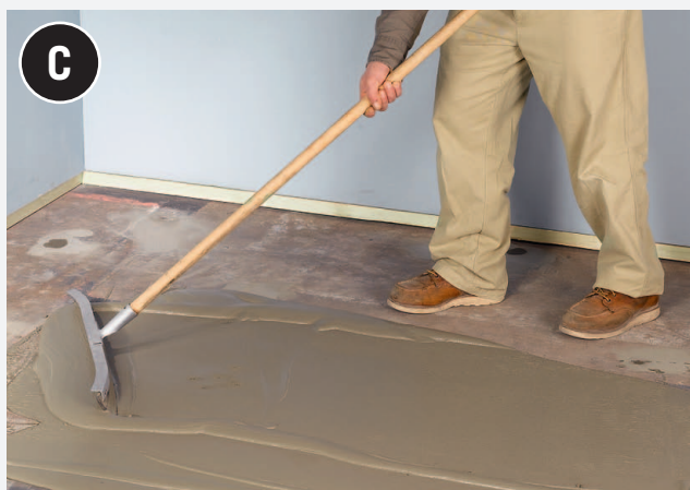
Spread the mixture across the floor evenly using a long-handled squeegee. Don't apply layers more than ½-inch thick. Let it cure for at least a day before walking on it.
