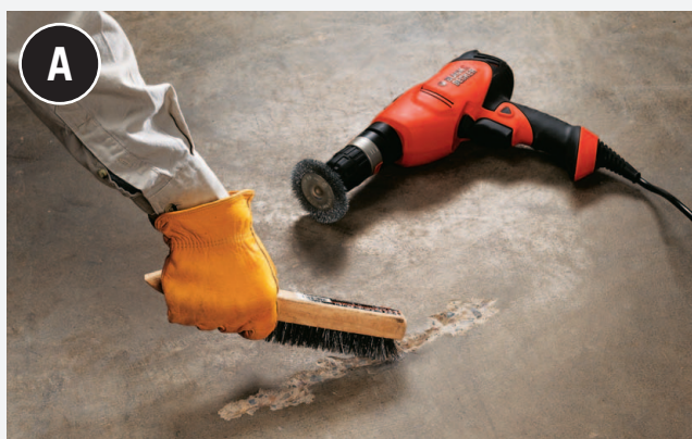
A Clean out the damaged area with a wire brush and/or a wire wheel attachment in a power drill.
