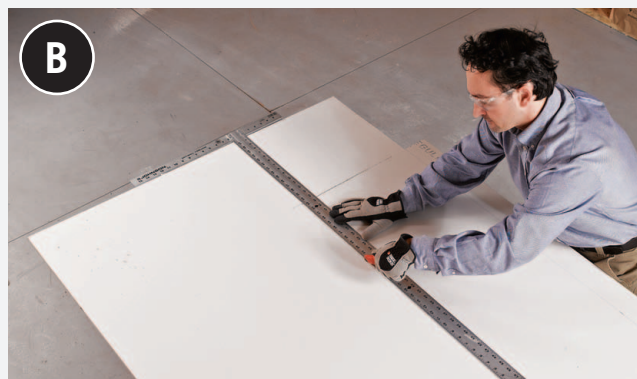
Use a utility knife and drywall T-square to cut drywall panels to fit.
