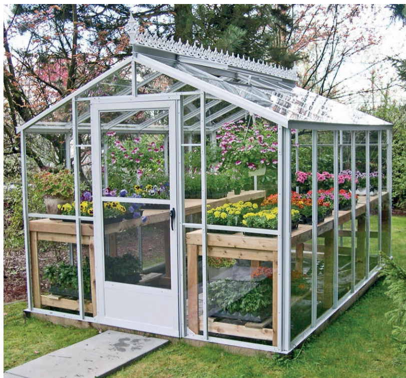
An upscale example of a handsome prefab , aluminum-framed greenhouse. Used with rubber gaskets and glass panels, this construction can easily withstand even high wind loads. The crest and finial are finished in long-lasting baked enamel. A crest like this, as well as adding flair to the greenhouse's look, also keeps birds from perching on the ridge—which in turn keeps the panels cleaner.
