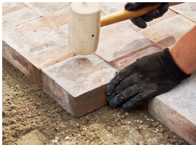
Concrete pavers set in sand offer a long-lasting, stable floor covering that breathes and allows for good drainage.
