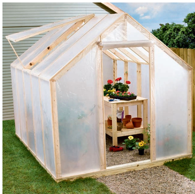
A pine frame with plastic glazing. This is a good option for a lightweight and inexpensive greenhouse that will be used for two or three seasons.
