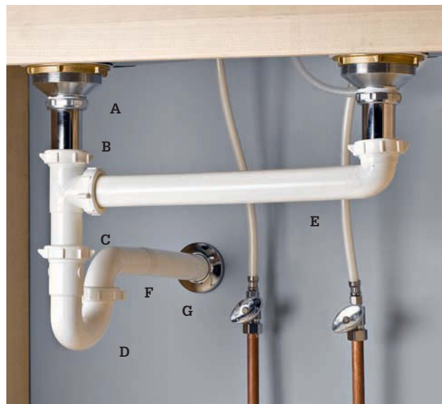
Kitchen sink drains include a strainer body (A), tailpiece (B), waste tee (C), P-trap (D), outlet drain line (E), trap arm (F), and wall stubout with coupling (G).
