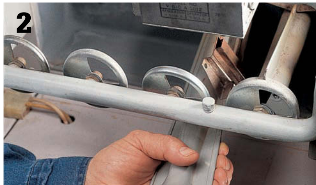
If a burner is difficult to remove , twist it carefully from side to side while lifting and pulling.
