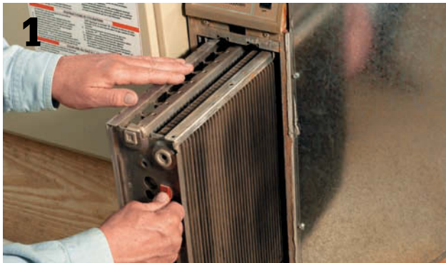
Clean electronic filters every month , then reinsert them in your furnace.
