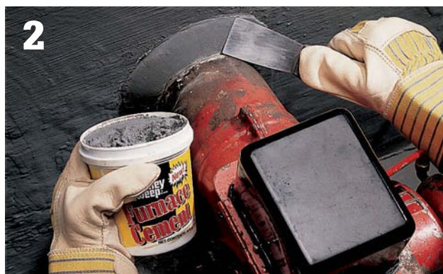
With a putty knife , apply refractory furnace cement to seal the leak.
