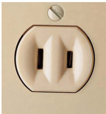
15 amps, 120 volts. Polarized two-slot receptacles are common in homes built before 1960. Slots are different sizes to accept polarized plugs.
