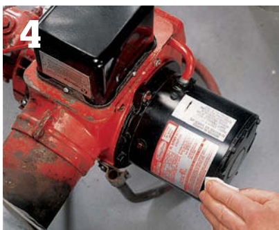
To prevent dust or dirt from getting in the motor while you add oil, clean off the surface with a damp cloth before opening the ports or cups.
