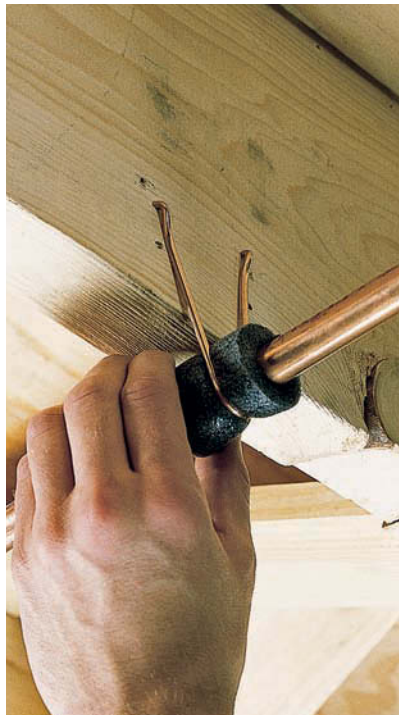
Loose pipes may bang or rub against joist hangers, creating noise. Use pieces of foam rubber pipe insulation to cushion pipes.
