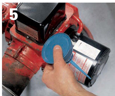
Add lubricating oil to the ports or cups. The motor housing may indicate what kind of oil to use.
