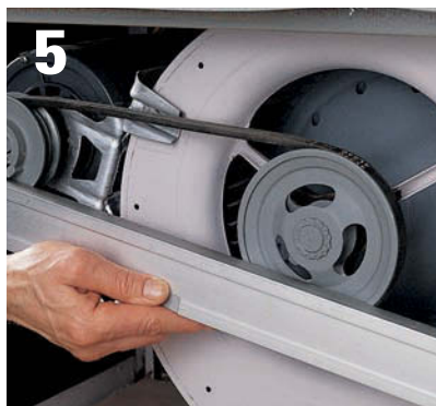
Check the pulley alignment , using a straightedge.
