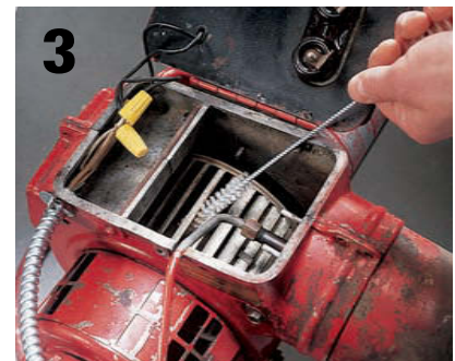
The blades on most blower fans are thin and hard to reach, so use a long brush carefully: a bent fan blade makes much more noise than a dirty one.
