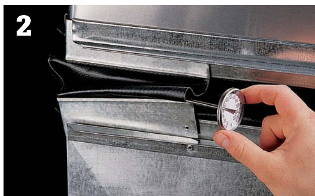
2 Check the temperature inside the supply duct and compare it with the temperature in the return duct.
