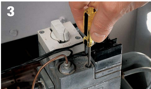
Turn the screw to adjust the height of the flame so it covers the top of the thermocouple.
