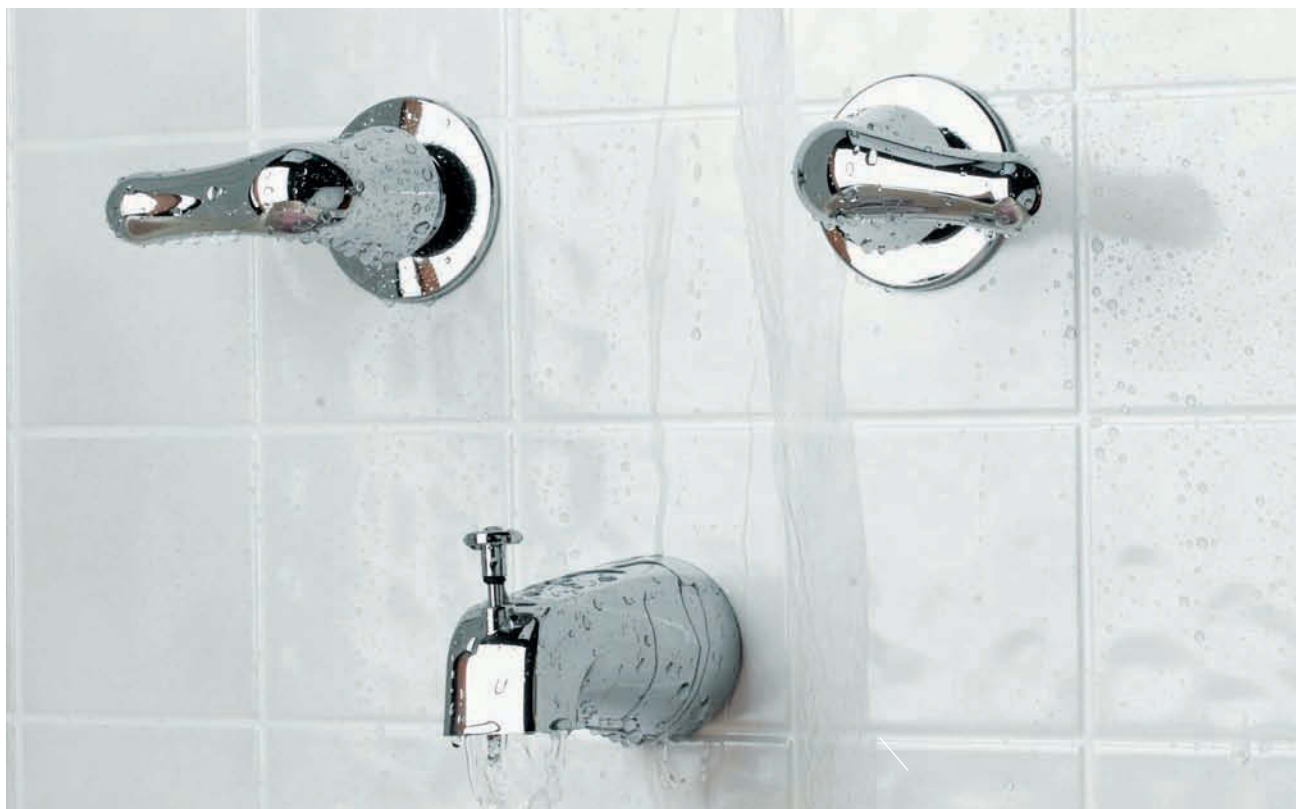
Tub/shower plumbing is notorious for developing drips from the tub spout and the showerhead. In most cases, the leak can be traced to the valves controlled by the faucet handles.
