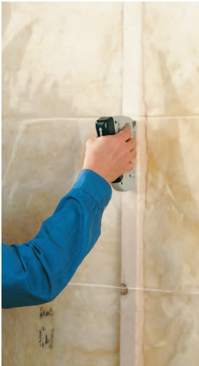
A moisture barrier consisting of 4-mil clear polyethylene sheeting can be stapled to framing members in damp areas before installing the cement board.
