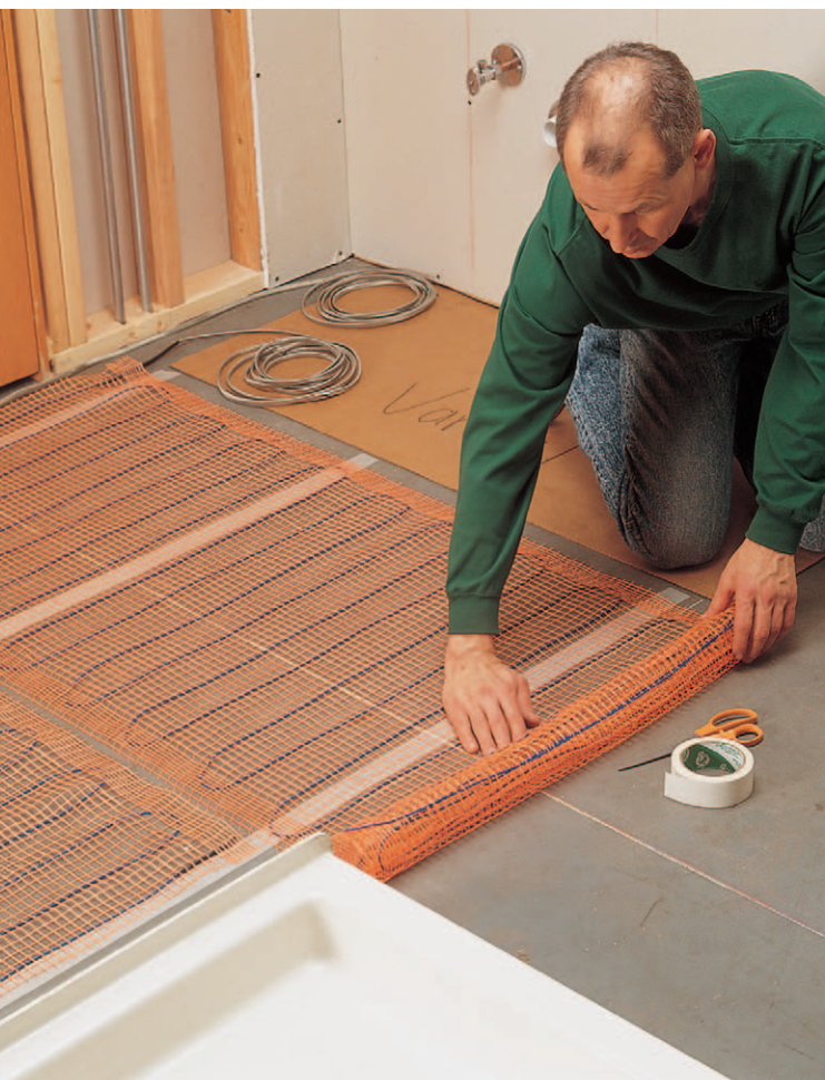
DIY radiant-heat floor systems are electric mats installed beneath floor coverings to warm your feet and heat your room.
