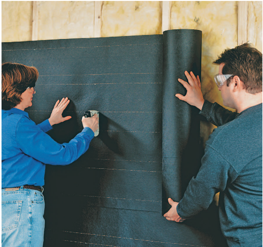
Asphalt roofing felt (15# building paper) can also be used as a moisture barrier behind cement board panels in damp areas.
