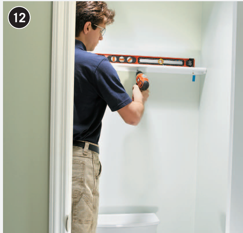
12 Paint the enclosure walls and add any additional elements, including paper holders, grab bars, and shelves or cabinets. The wall area behind the toilet tank is a good spot for installing shallow shelving, but keep it at least 3' above the tank lid.
