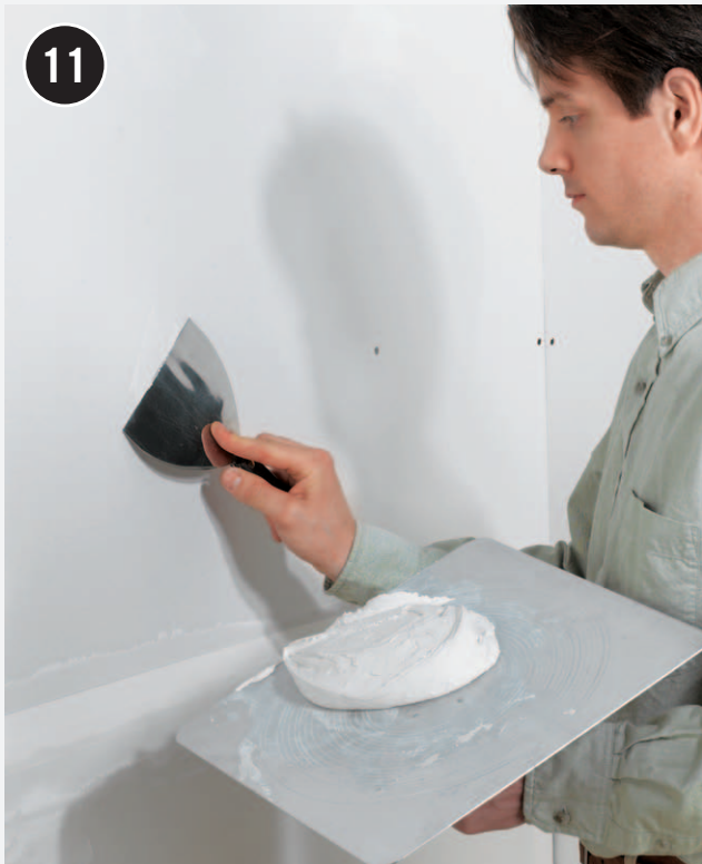
11 Finish the drywall surfaces with tape and joint compound. Work as neatly as you can to minimize sanding. Seal the new drywall with drywall primer before you paint.
