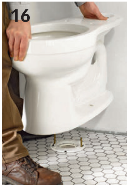
16 Install the toilet after trimming the closet drain pipe to the correct height. Hook up the water supply to the fill valve and then test the operation. Drain times can be a bit slower in basements, and flushes may be weakened slightly by the shallowness of the drain line slopes.
