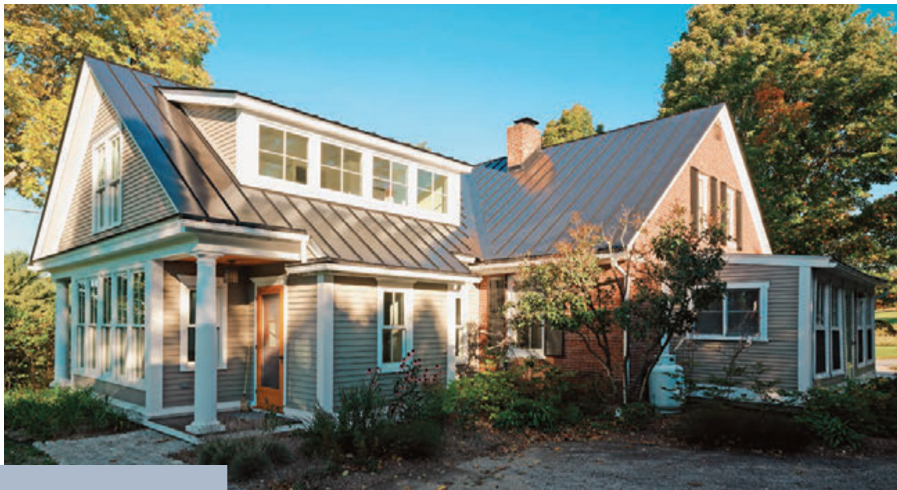
Side view of completed wing addition
