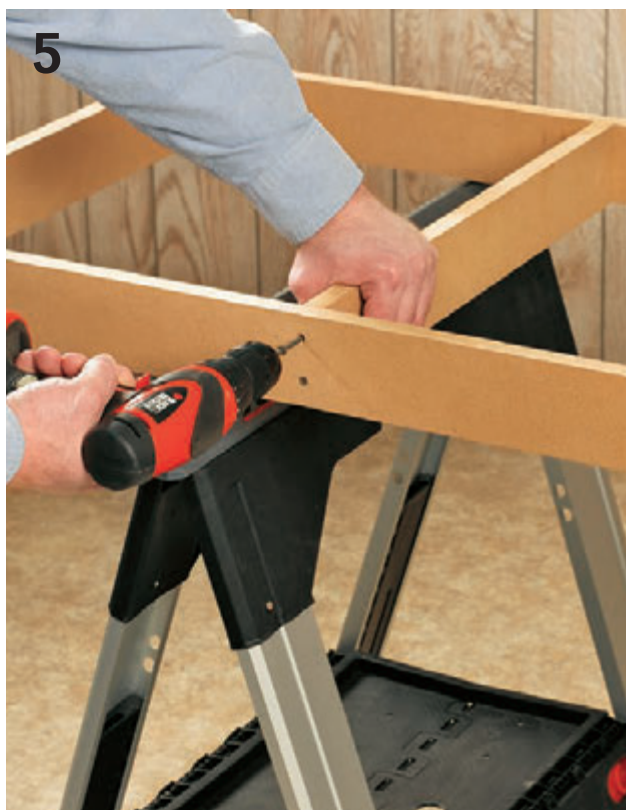
Assemble the curb members into a ladder-like frame and secure the butt joints with glue and screws driven through pilot holes.
