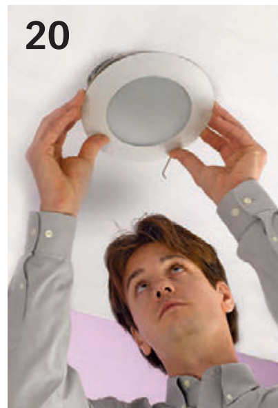
20 Attach trim kits and escutcheons to light fixtures and vent fans. Add switch plates and receptacle covers, too. Test all fixtures.
