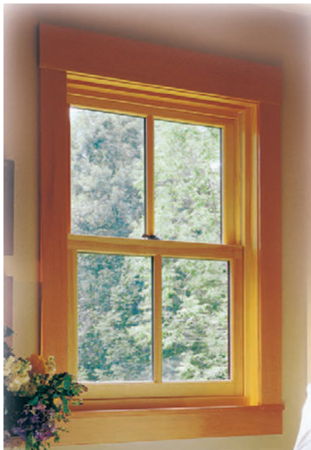
The window stool and apron give the window a finished appearance while offering the practical advantage of a window sill.
