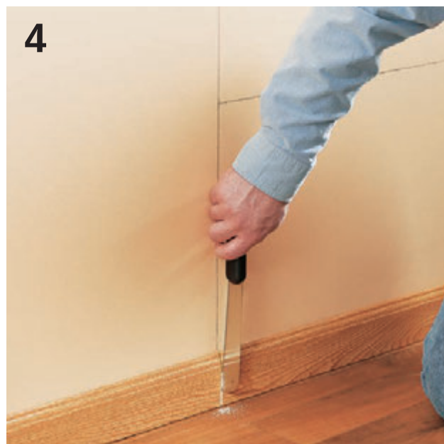
Because a pull-type saw requires almost zero clearance at the bottom of a cut (where it would hit the floor in this application), it's great for removing the base molding so the cabinet carcasses fit tight to the wall.
