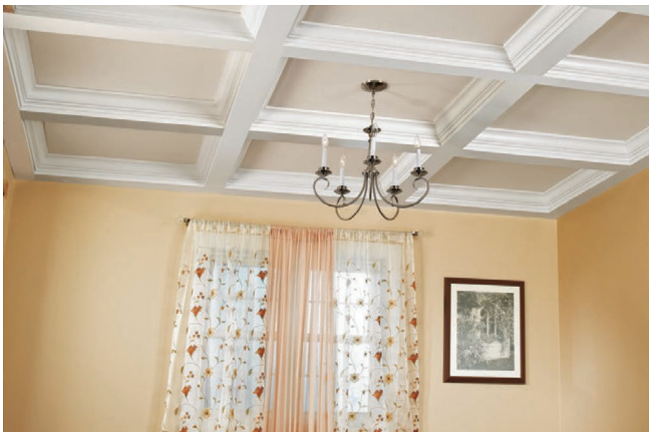
The rich architectural appeal of a coffered ceiling can be achieved with some strips of MDF and a little crown molding.
