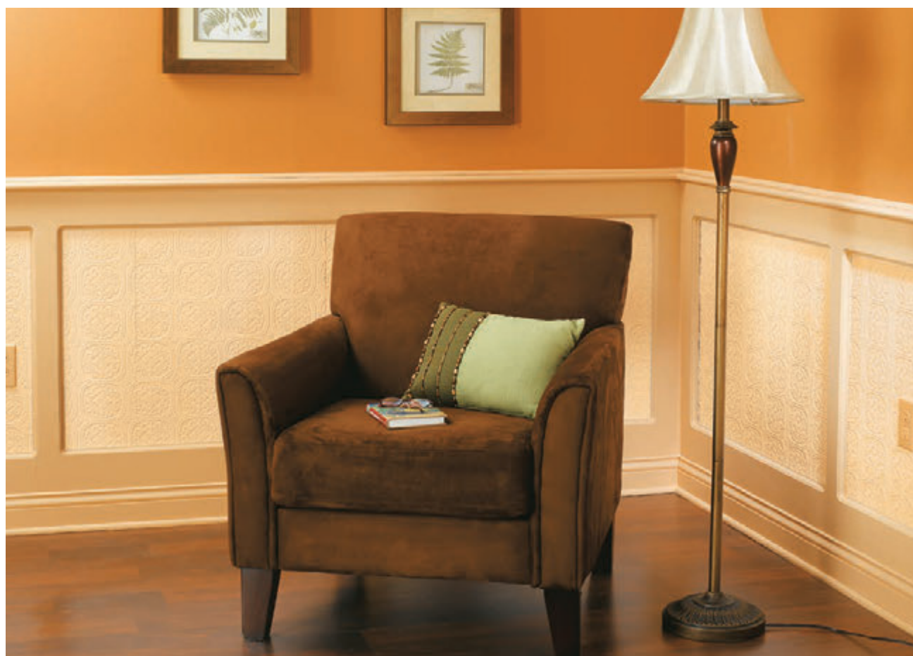
These wainscot frames are cut from full sheets of MDF, so they require virtually no joinery.
