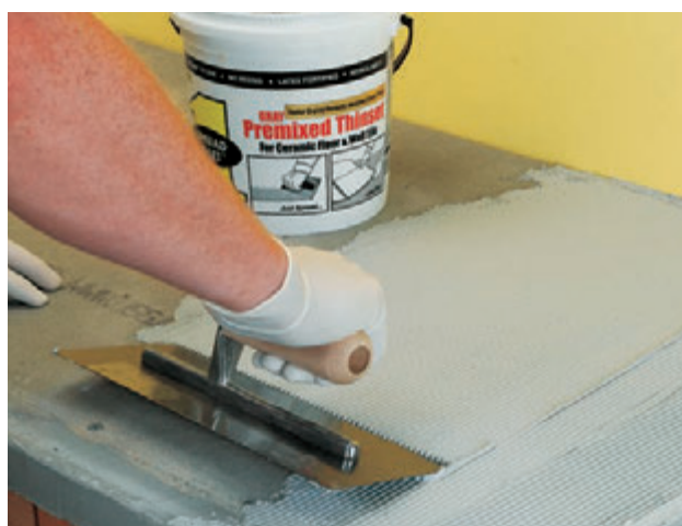
Tiles are set into a bed of thinset mortar troweled onto a cementboard or tilebacker subbase.
