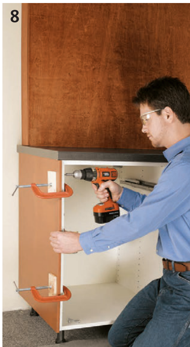
Attach the wall and base cabinet side panels. Clamp the panel to the cabinet side and drive 1" screws through the inside face of the cabinet side. Then install the toe-kicks.
