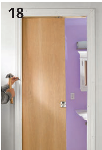
18 Hang the entry door and install trim around the door as well as a baseboard trim. You may find it easier to paint or finish the door and trim before installation.
