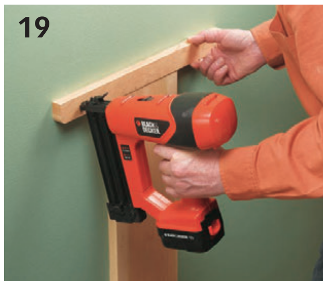
Attach a 1 × 2 stop block for the lift gate to the wall directly above the wall-mounted end panel.
