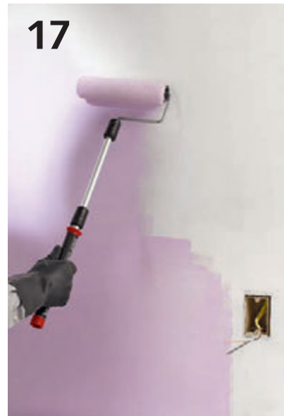
17 Paint the walls and ceiling using a paint with a mold-resistant additive. Paint the ceiling first. For bathrooms, choose a washable, semigloss paint.
