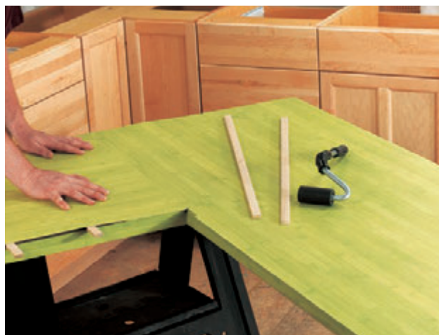
Plastic laminate is bonded to a particleboard subbase with contact cement.
