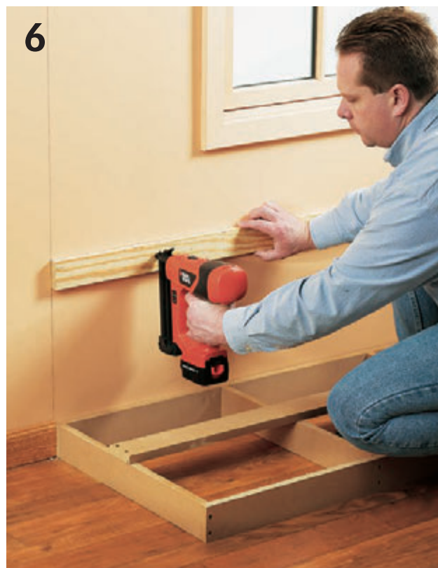
Attach a ledger for the back edge of the seatboard to the wall, using panel adhesive and screws driven at stud locations. Tack the ledger in place and then reinforce with wood screws driven at stud locations.
