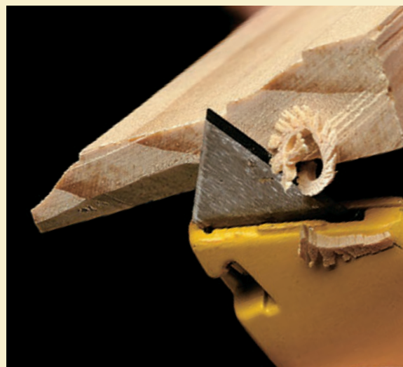
Back-cut the ends of casing pieces where needed to help create tight joints, using a sharp utility knife.
