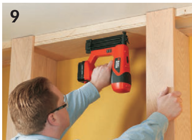
Attach a shelf board at the top of each bay to conceal the framework attached to the ceiling.
