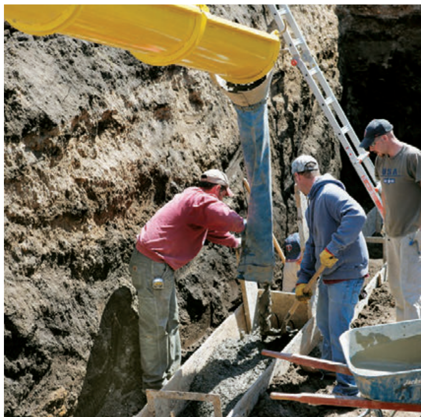
A concrete footing provides a flat, sturdy surface on which you can stack concrete block foundation walls or pour concrete walls.
