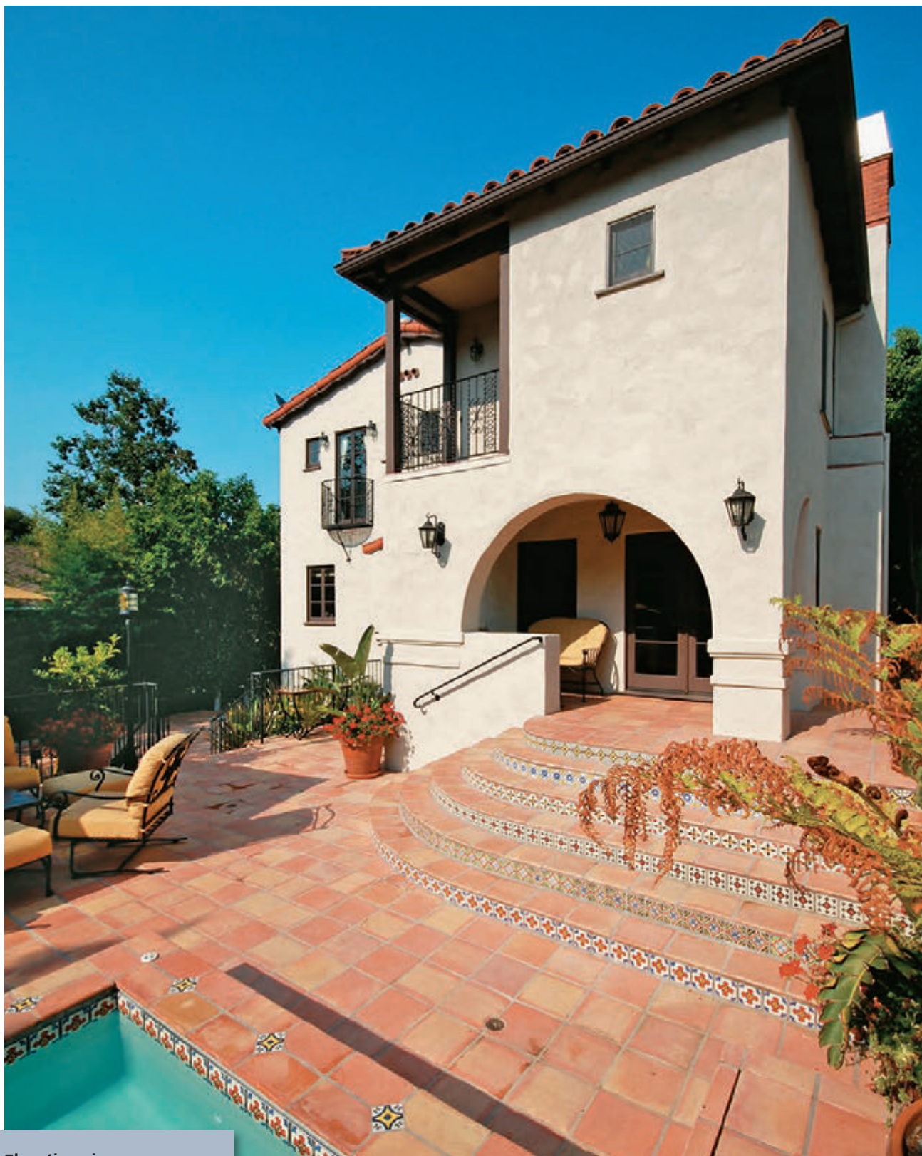
Elevation view of completed two-story bumpout
