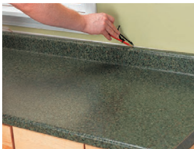
Post-form countertops have a laminate surface that is applied at the factory.
