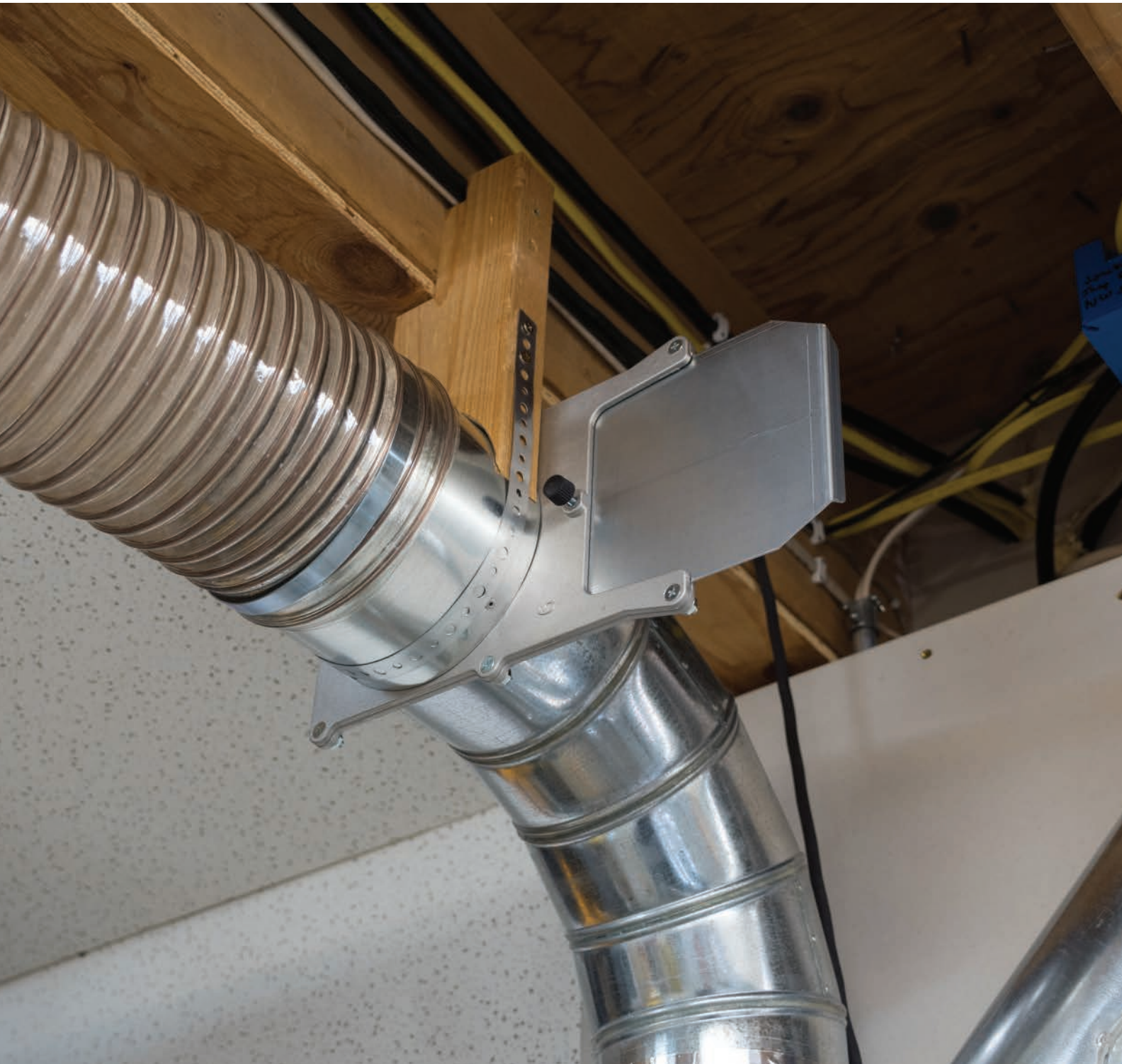
In a central collection system, suction is maintained by opening and closing gates to individual tools.
