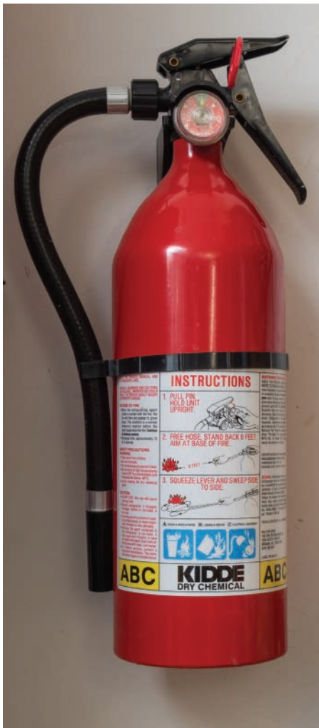
An ABC fire extinguisher will extinguish most types of fires. Be sure to mount it in an obvious, easy-to-reach location.
