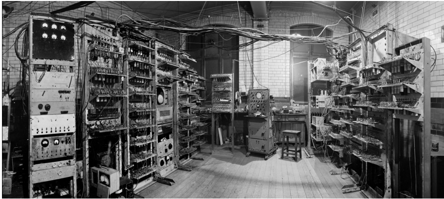
Full view of the Manchester Baby, a composite of 20 photos taken by Alec Robinson on 15 December 1948; for an annotated version, visit history.cs.manchester.ac.uk/?action=getSet&set=SET0002
